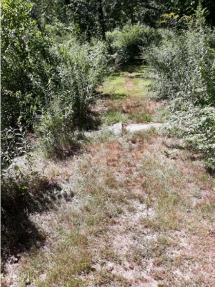
Northern crossing with culvert, stabilized soil conditions on approaches
