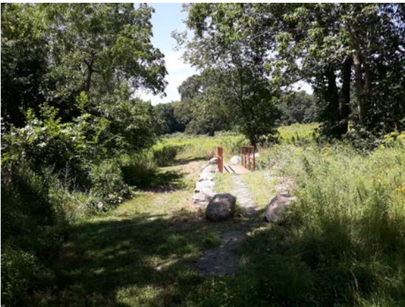
Central crossing with bridge and stabilized soil conditions. Stone ford at left of bridge.
